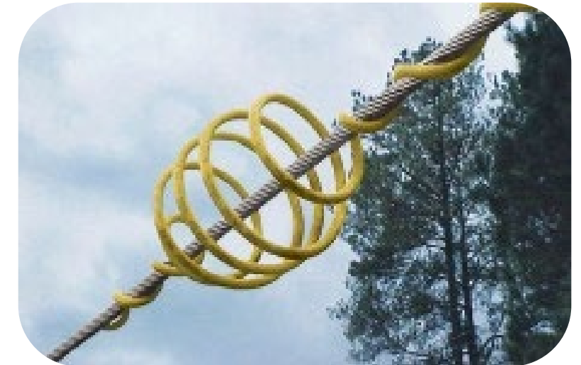
Swan-Flight Diverter – Visible only to swans and humans
